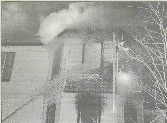
House on South 9th Street was extensively damaged by fire Sunday night.
